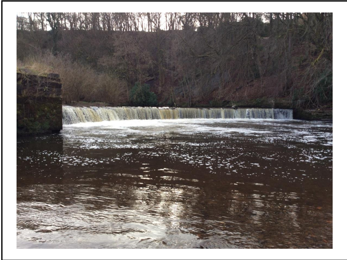
Figure 3.3: Photograph of Stringer's weir along the river Goyt
