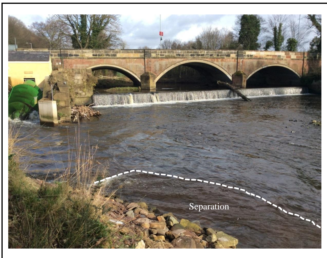
Figure 5.12: Photograph of the confluence below the hydro showing evidence of an area of separation towards the bank
