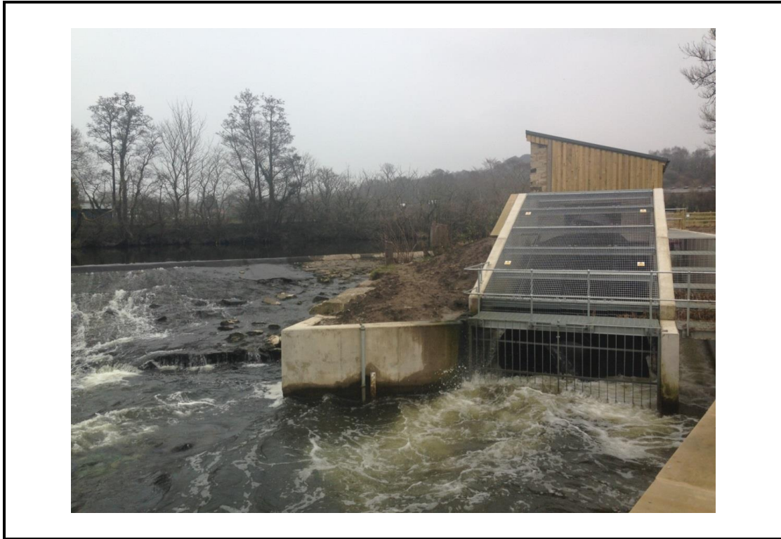
Figure 2.11: Photograph of turbulence below the turbine at a low head 'on weir' scheme in the River Calder, UK
