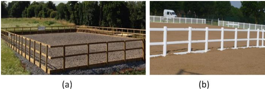
Figure 1.2: Image of equestrian fence: (a) timber and (b) PVC
