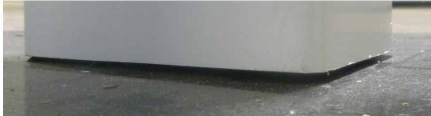
Figure 5.25: Image showing separation between the base of the centre PVC post and steel plate when a load of 600 N was applied at the top of the former (Node C)
