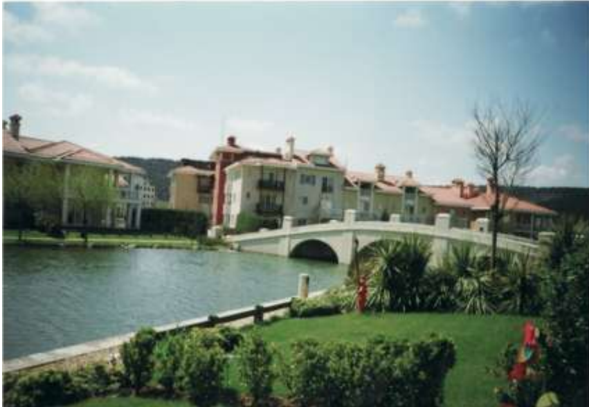
Fig 6.1.3.2: Istanbul Istanbul, artificial lake and bridge, which was built similar to a summer resort in France.
