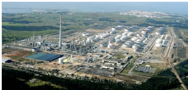
Fig. 2. GALP oil refinery.
