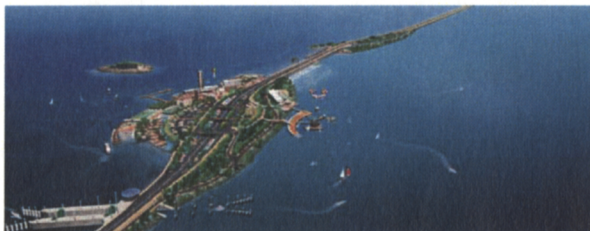
Bird's eye view of Sihwa tidal power plant to be completed in 2009 © DAEWOO
