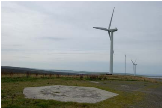
Evidence:base of wind turbine at Burgar Hill.
