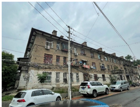
Figure4-6. The Staff Dormitory Building(By the author)
