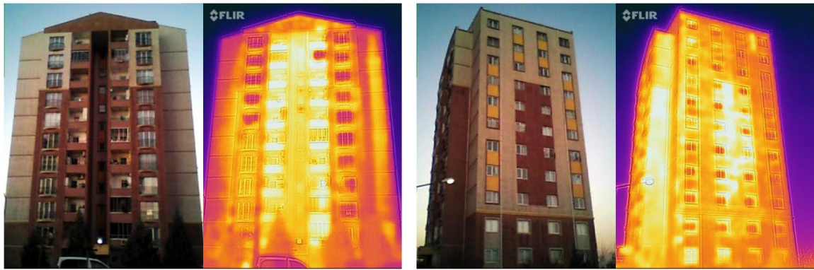
Figure 11. Exterior wall temperature on the southwest (left) and southeast (right) façades of Block 3 in TOKI Etiler in December
