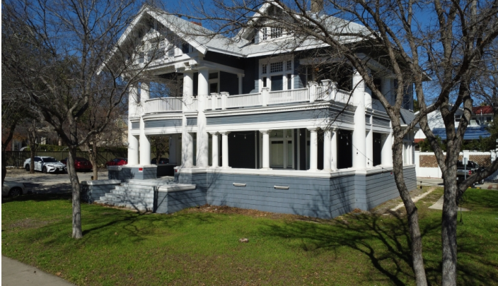
Figure 2. The Kelso House after the exterior restoration, as viewed from the southeast orientation. Source: Assaad Akle, 2023.
