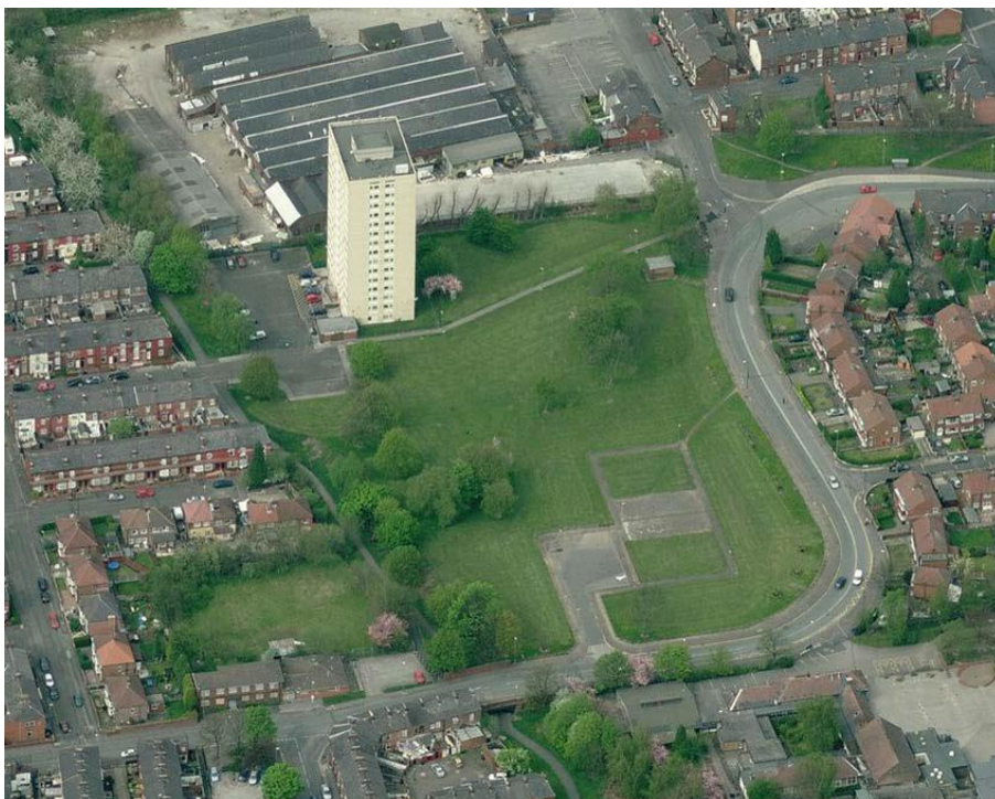
Figure 7.16: Aerial view of Gorton Mill site, Abbey Hey, 2019. SOURCE: Google maps
