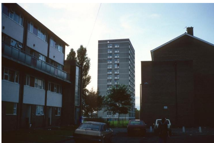
Figure 7.42: View of Abbey Court from Longford St, c.1987, with maisonettes (now demolished) SOURCE: Tower Block.aca.ed.ac.uk, The University of Edinburgh
