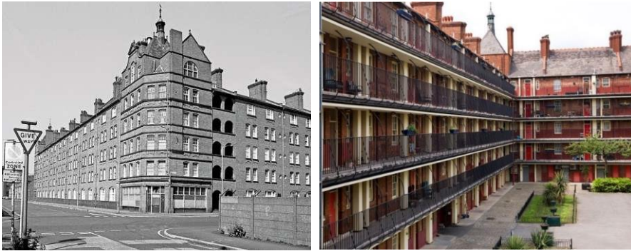
Figure 7.33: Victoria Square Building, 1889 – 1894, Oldham Road, Ancoats, Manchester. SOURCE, LEFT: Manchester Victorian Architects.org.uk , RIGHT: Historic England, Ancoats.
