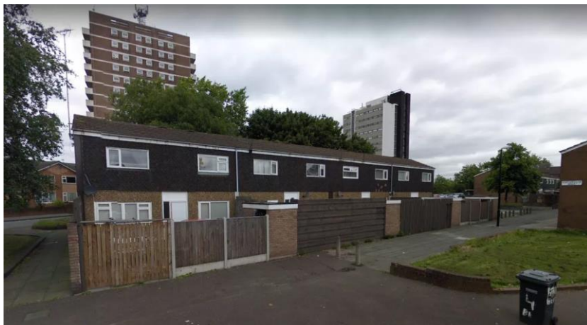
Figure 7.40: Wenlock Court in background and the filming location for the Chatsworth Estate . SOURCE: Liverpool Echo (19.11.2022)
