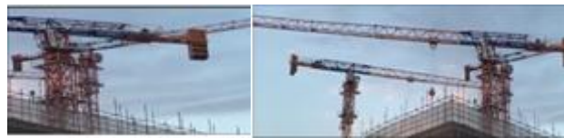
Figure 13: Example of two tower cranes overlapped in one image
