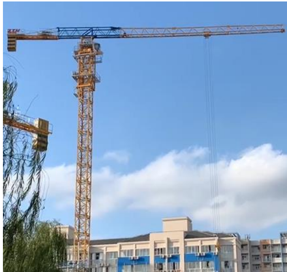
Figure 2. Physical entity of the QTZ80 tower crane
