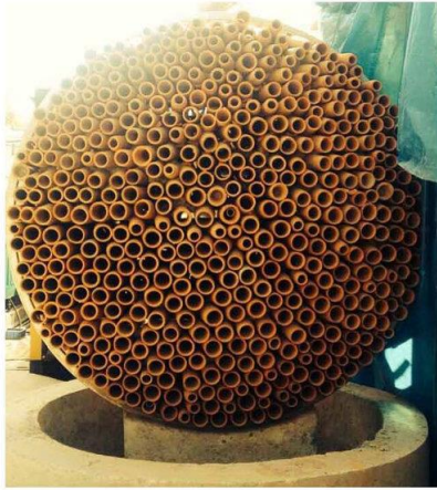
Figure 7. Terracotta low-tech air-conditioner (Ant Studio, 2017).
