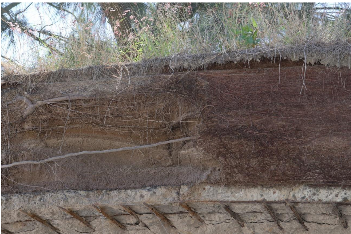
Figure 3: A photograph showing layers of sediment and ash deposited on top of a building's roof in Montserrat. Photography credited to Professor John Quinton.
