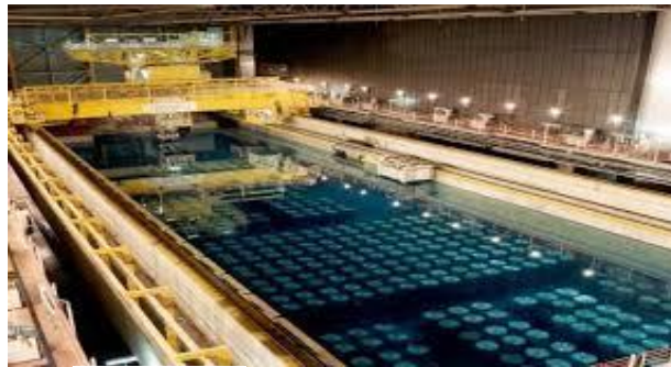
Figure 2.5: Receipt of spent fuel and interim storage at THORP [30] (reproduced with permission from reference [30], copyright 2015 Sellafield Ltd.).
