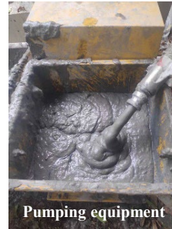
(c) Pumping concrete
