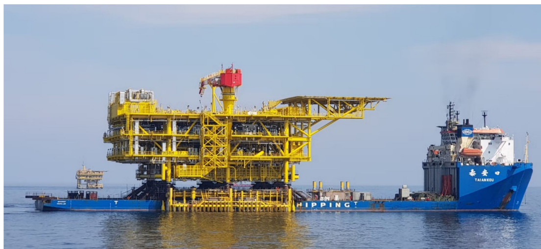
Figure 12. Jacket platform topside being transported floatover installation towards platform integration (Courtesy: Saudi Aramco).
