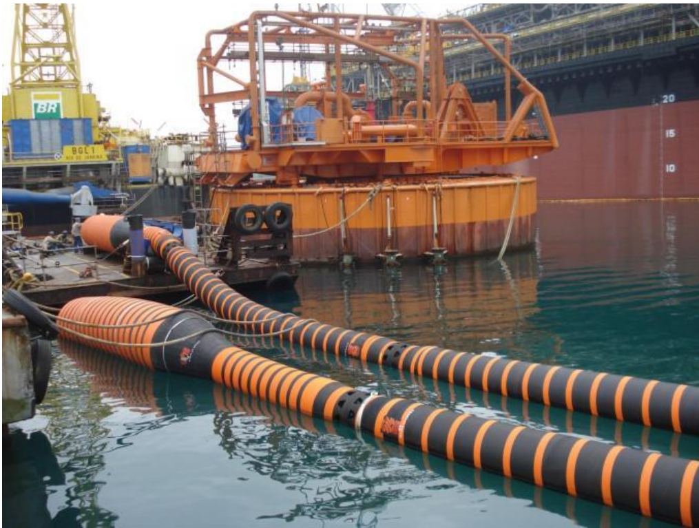
Figure 19 Installation of floating hoses for a CALM buoy in offshore Brazil (Courtesy: BR)
