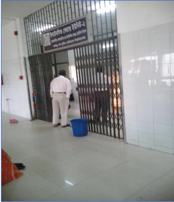
Picture 5 The collapsible gate at UTH
