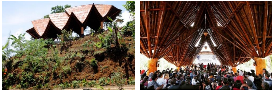
Figure 16: The completed bamboo church building in 2019 (ASF-ID, 2019)
