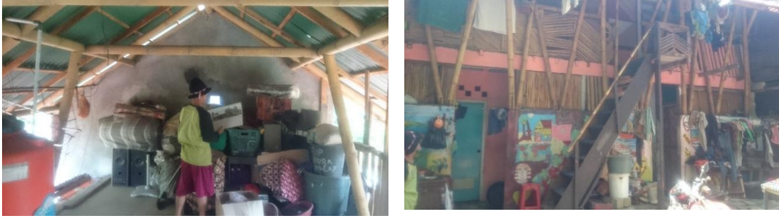
Figure 10: Several changes in the post-construction phase (Setiawan, 2017)
