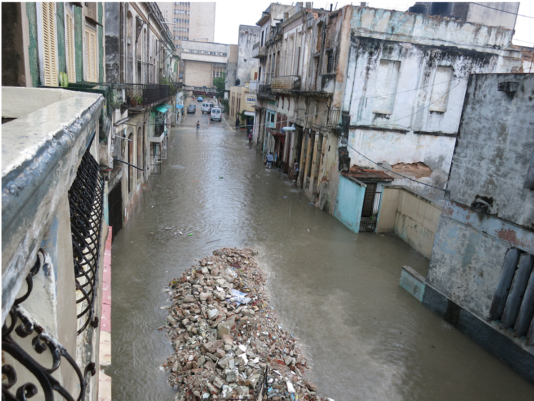
Top to bottom: Smoke billows from the hospital incinerator chimney in the next block; Rubble from a building collapse forms an island when the street floods during heavy rain, Central Havana, 2016.
