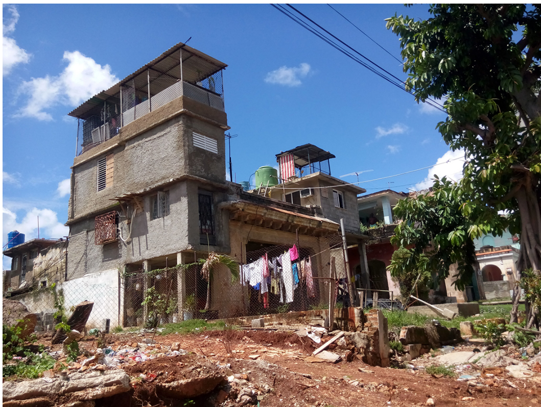
A flat reinforced concrete roof is much prized for the possibility to build extra floors, Playa, Havana, 2017.
