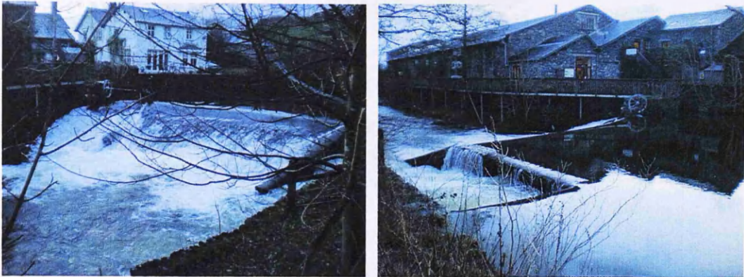
Figure 6-13 Weir in Staveley
