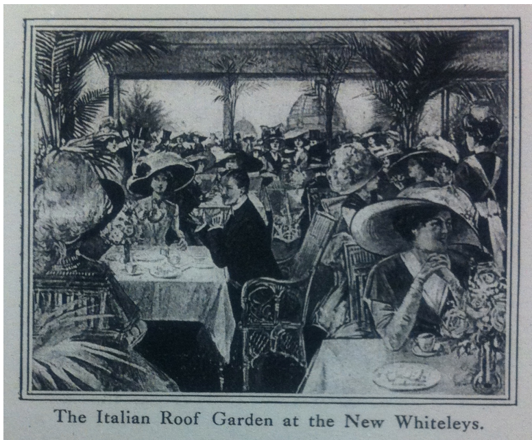
Figure 7.2 – The Italian roof garden at the new Whiteley’s. Souvenir of the Laying of the Foundation Stone of the New Premises of Wm. Whiteley Ltd. Queen’s Road. October 1910: 18. WA 726/248.
