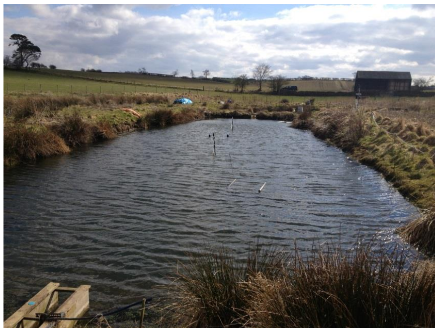
Figure 2.4 The shallow cell of the wetland looking South (upstream). The outlet flume is visible in the bottom of the picture, with the in-wetland wells in the centre and the middle flume visible in the distance.
