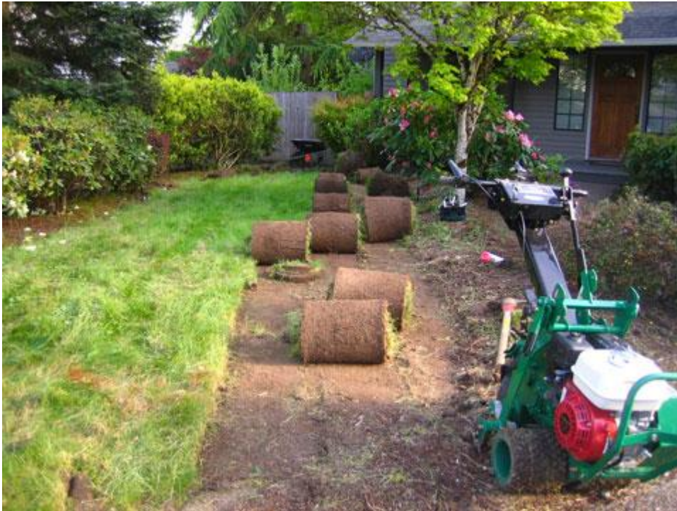
Figure 15. Sod cutter used in residential setting (Evergreen 2015).
