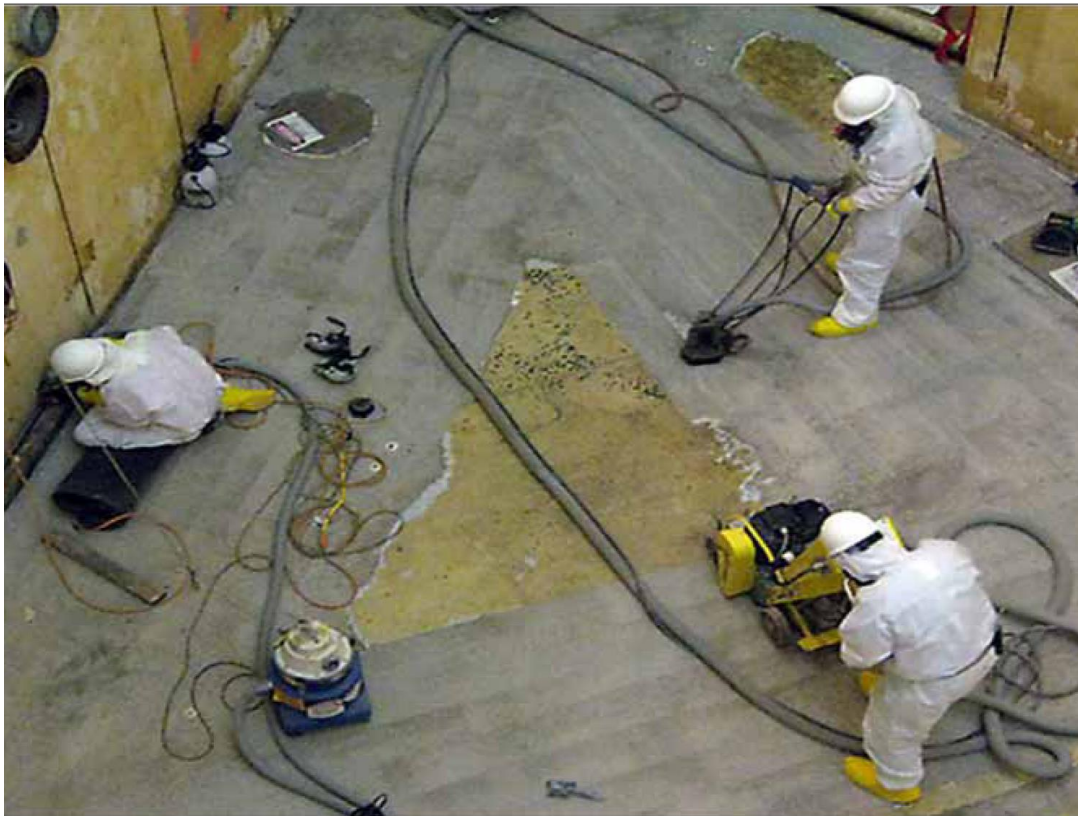
Figure 8. Scabblers being used at the Plum Brook Research Reactor (Boing 2015).
