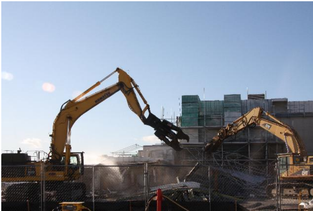
Figure 13. Nuclear facility demolition at the DOE Hanford Site (Nuclear Street 2012).
