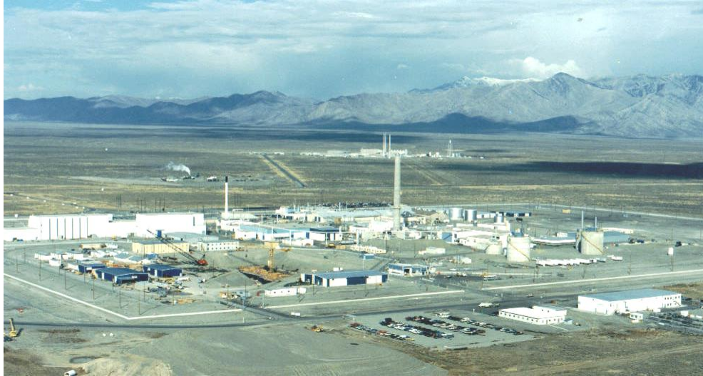
Figure 5. Idaho National Laboratory nuclear fuel reprocessing facility.
