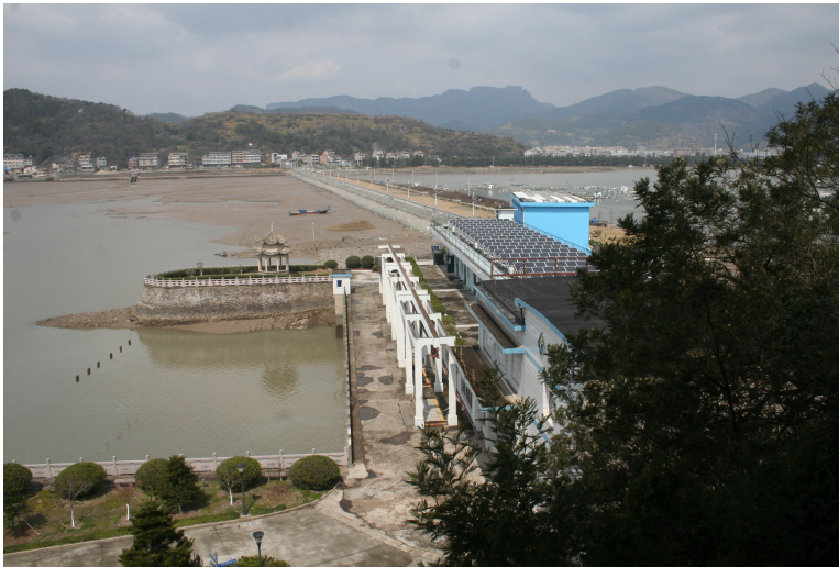
Figure 6 - Jiangxia tidal barrage (Maritime Tidal Energy, 2010)
