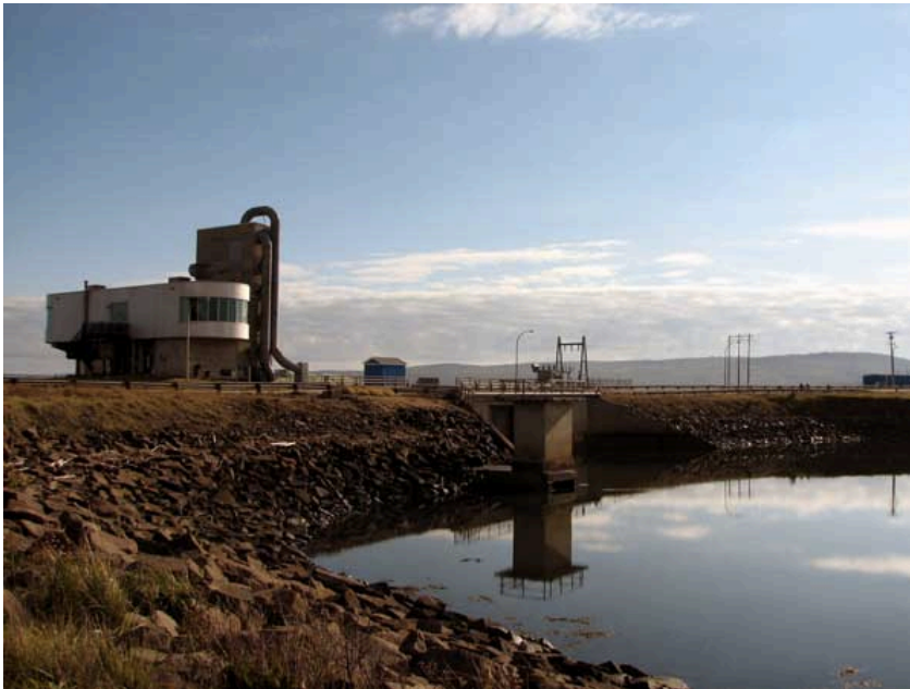
Figure 5 - Annapolis Tidal Barrage plant (Annapolis Valley Vacation, n.d.)
