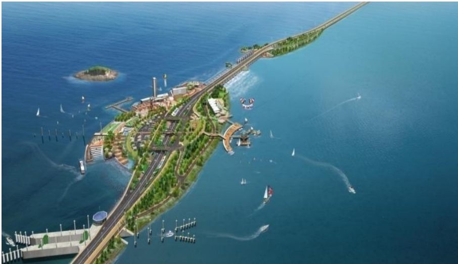
Figure 3 - Lake Sihwa tidal barrage (Aggidis, 2010)
