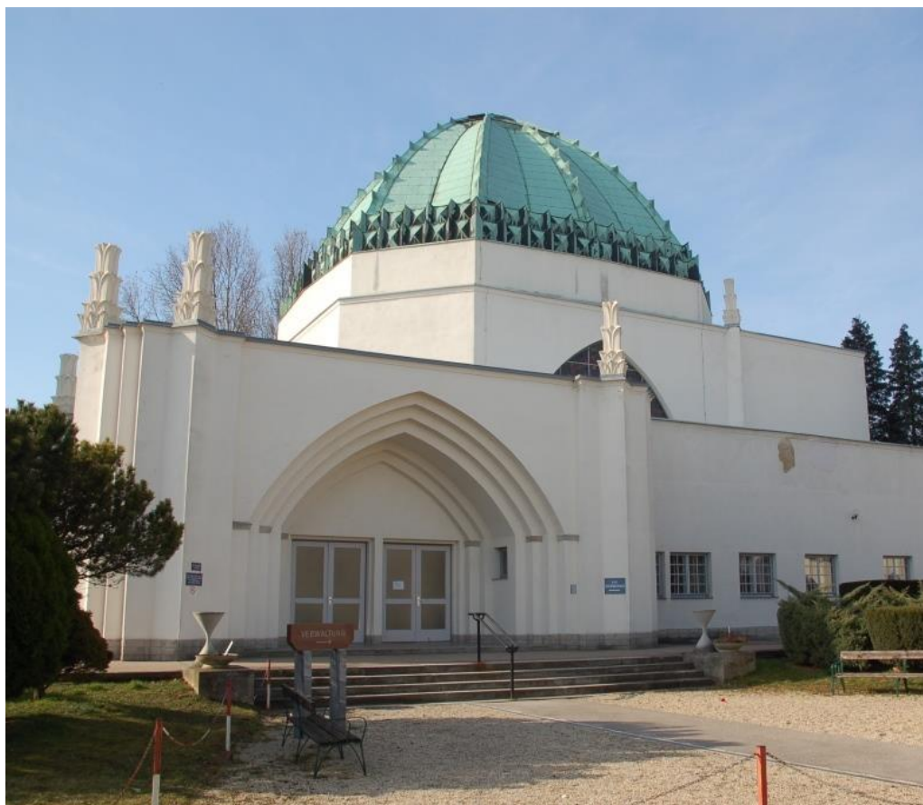
Figure 3.5: Restored beit tahara at Tor IV.
