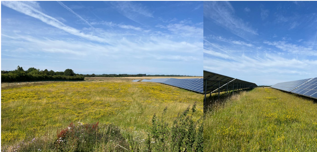
001. Images of Westmill Solar Park, Oxfordshire from the boundaries (left) and between a row of the solar array (right). Ben Secker
