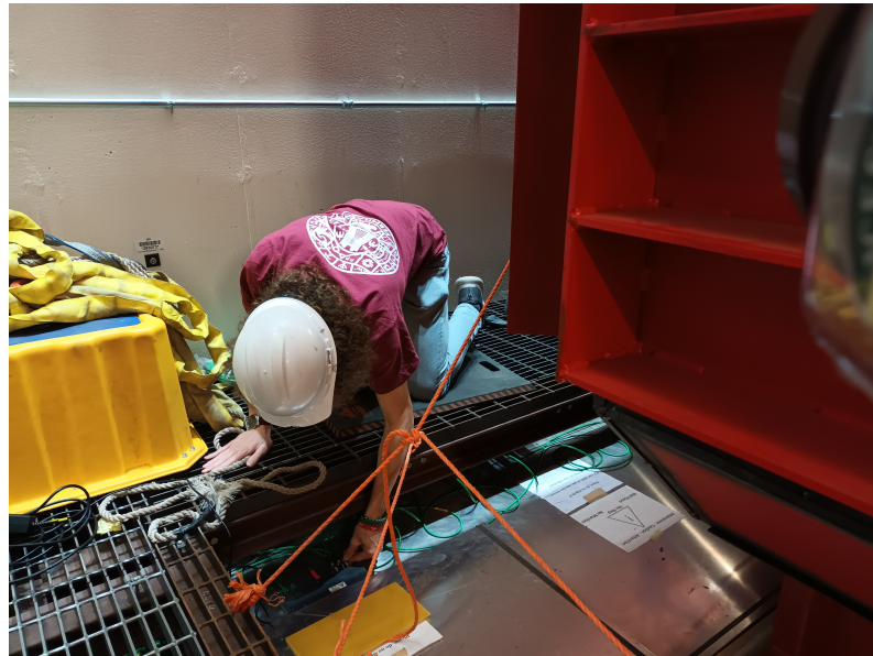
(b) Me installing cables in the CRTb setup, February 2023.
