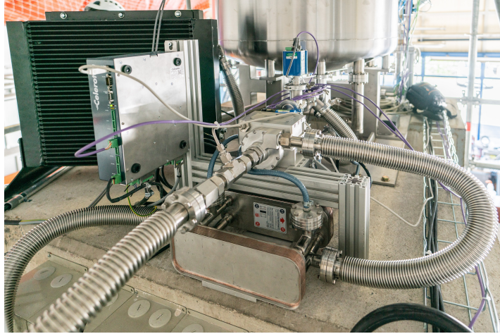
Figure 6: Picture of the Celeroton compressor and the water/glycol-cooling as installed at CERN.
