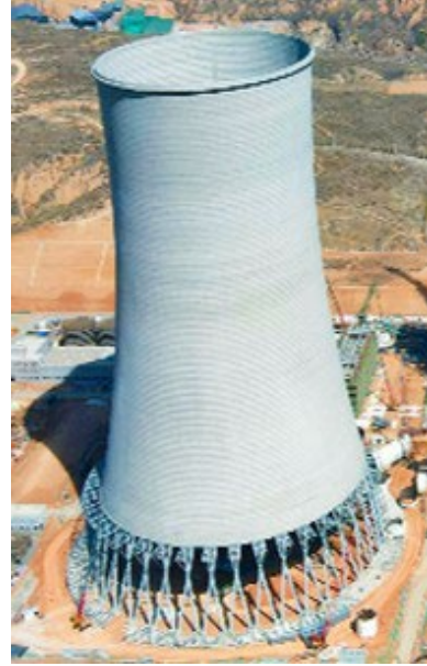
b). Cooling tower of power plant
