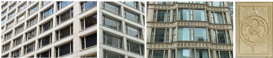
Figure 5: Horizontal Chicago-style windows and terra-cotta (Personal collection of Egemen Deniz Bahar).
