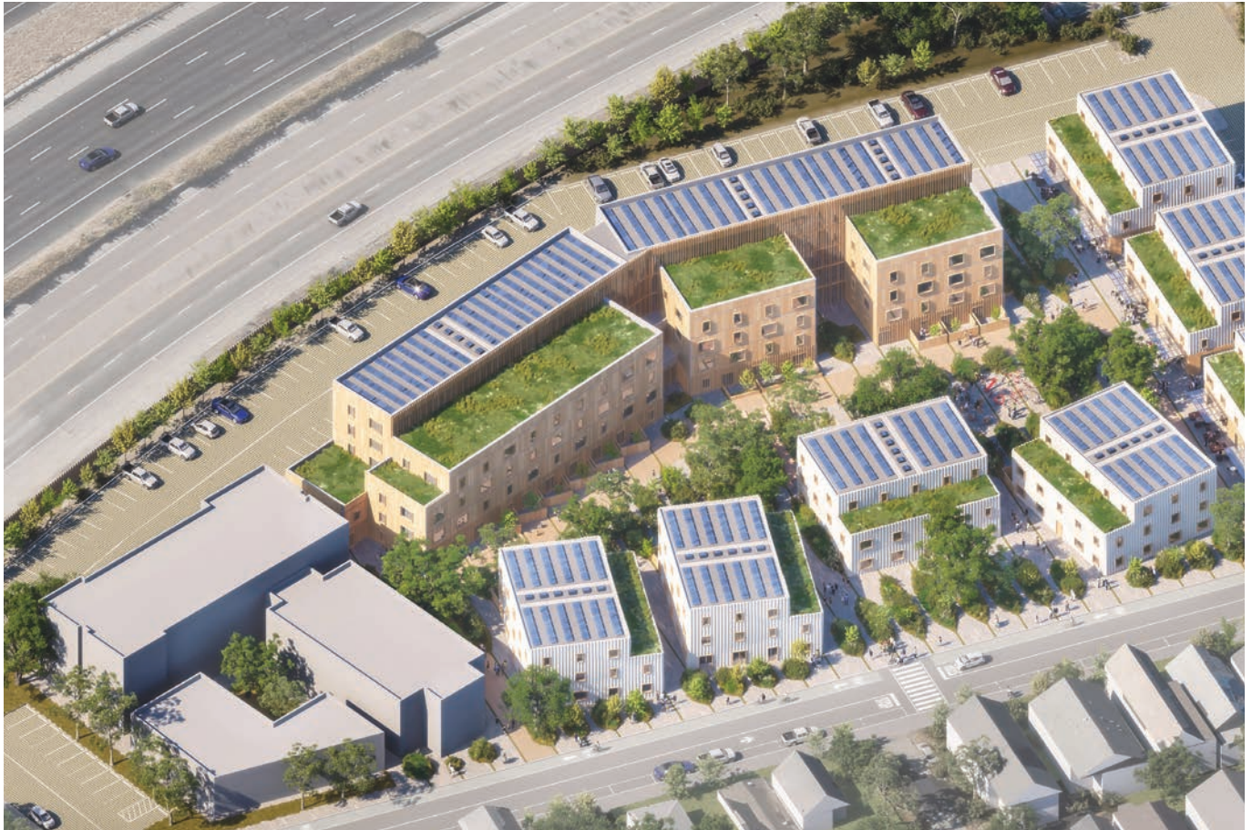
The Phoenix will be built at about half the cost, time, and carbon footprint of a typical multi-family building in the San Francisco Bay Area. Image courtesy of Autodesk.
