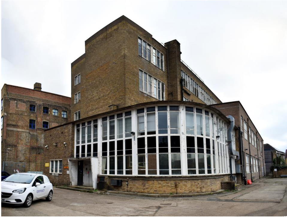
Figure 8: The 1949 Chiswick Telephone Exchange with a later extension at the rear. (Source: author's own)
