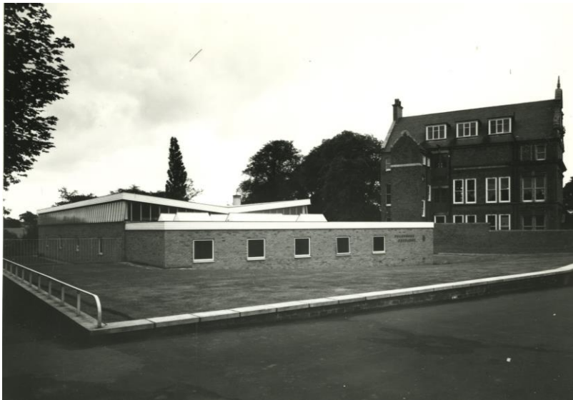
Figure 5: The 1960 Altrincham Telephone Exchange, with the original NTC Telephone Exchange in the background. (Source: BT Group Archives)
