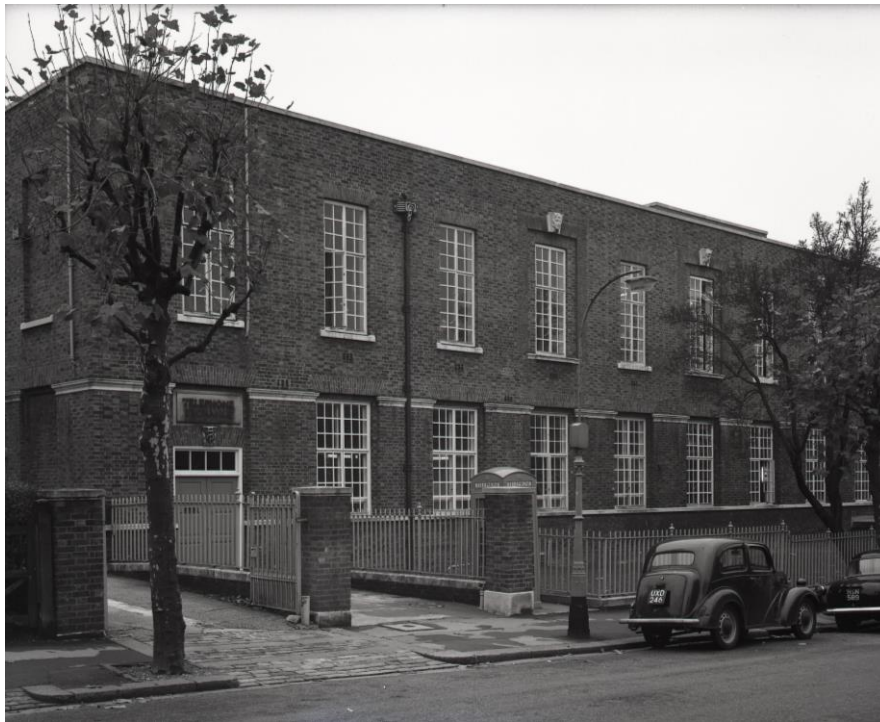
Figure 4: The Highgate Wood Telephone Exchange, where Britain's first electronic telephone exchange opened in 1962. (Source: BT Group Archives)
