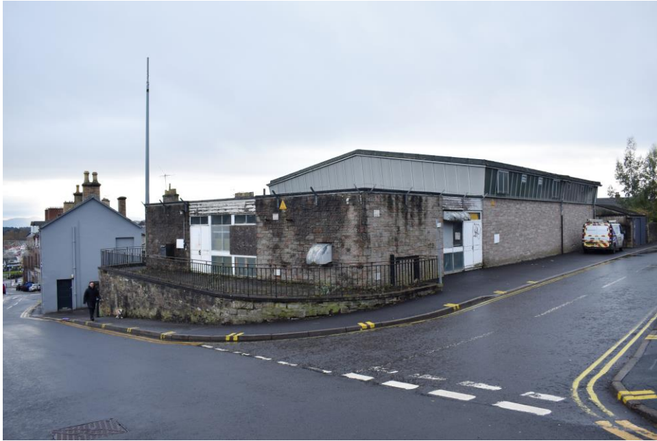
Figure 6: The Blairgowrie Telephone Exchange, clad in stone to suit the local vernacular. (Source: author's own)
