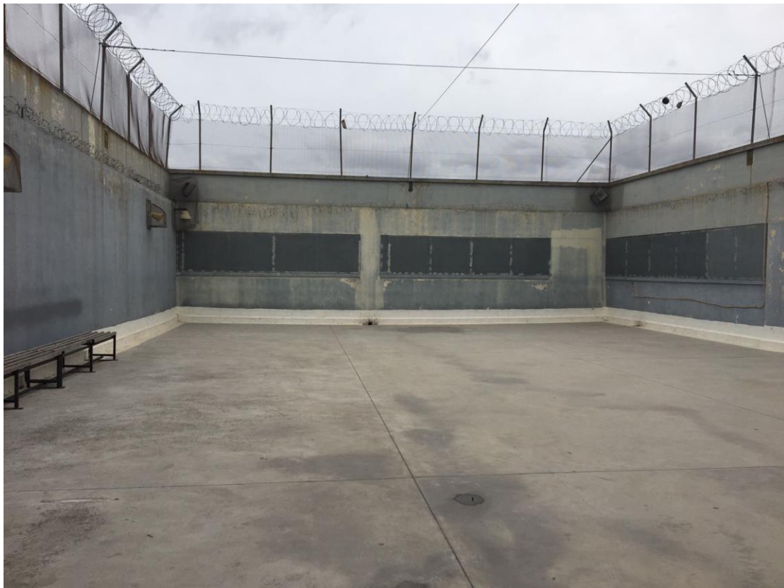
Figure 7: The outside area of the Petrou Ralli detention centre
