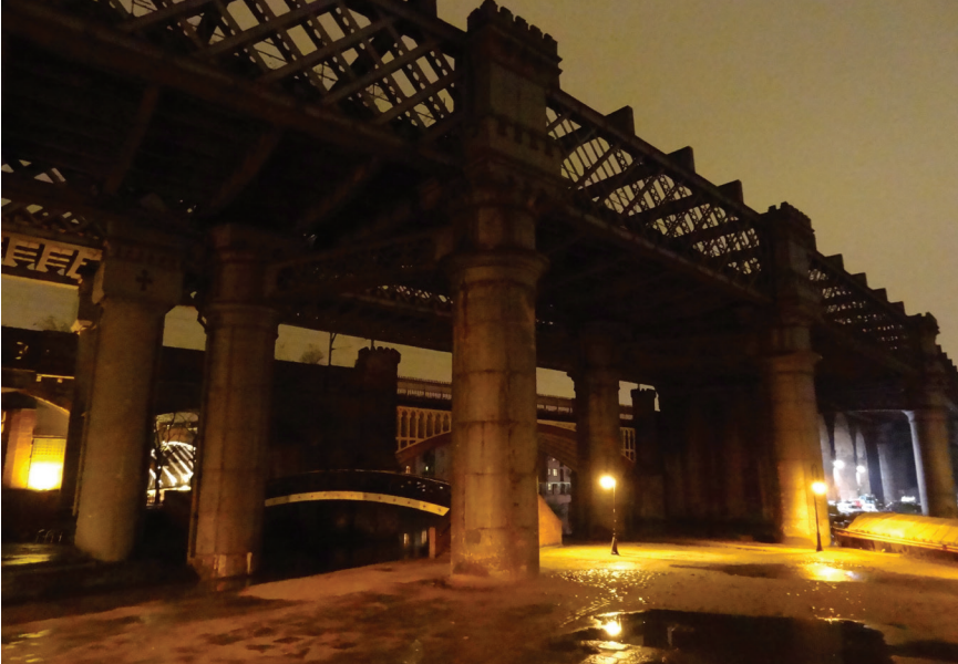
Figure 3. Sodium lamps, Castlefield, Manchester, 26 May 2016. © Nick Dunn. The quality and quantity of this form of artificial illumination was commonplace in many cities by the second half of the twentieth century.
