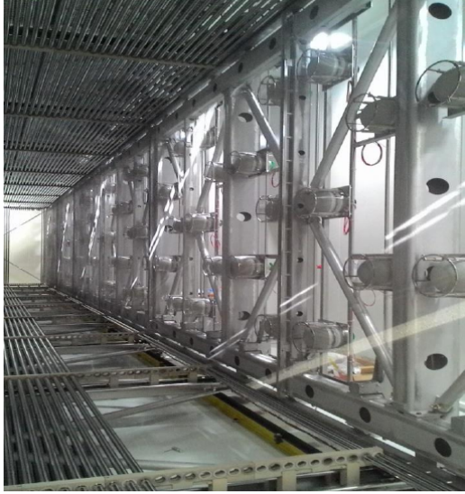
Figure 3. The new ICARUS PMTs mounted behind the wires of one TPC.
