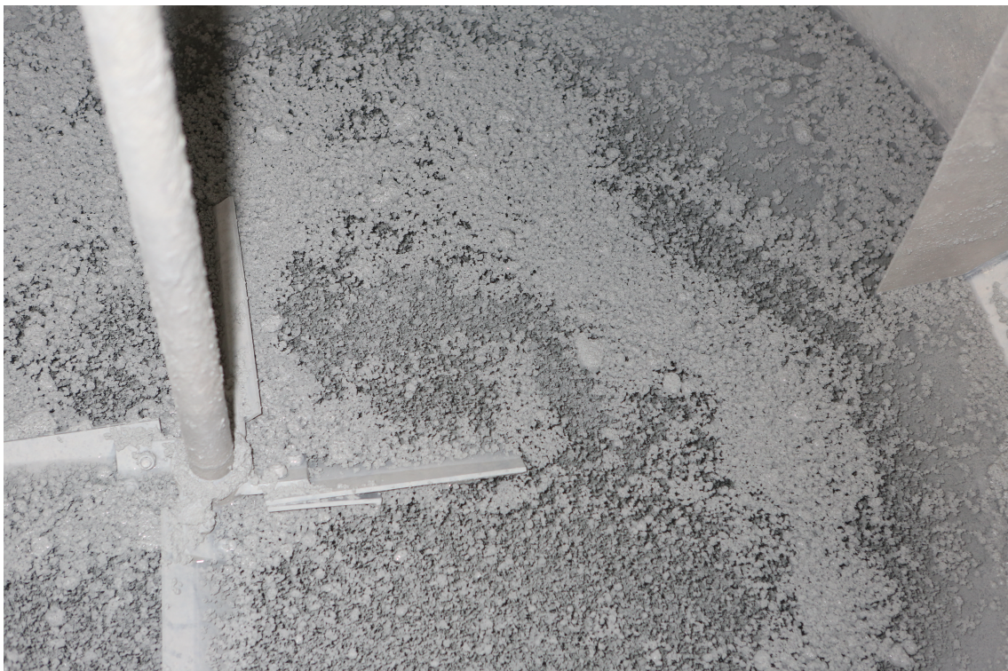
Figure 57: Flocs at Crown Paints Darwen effluent plant.
