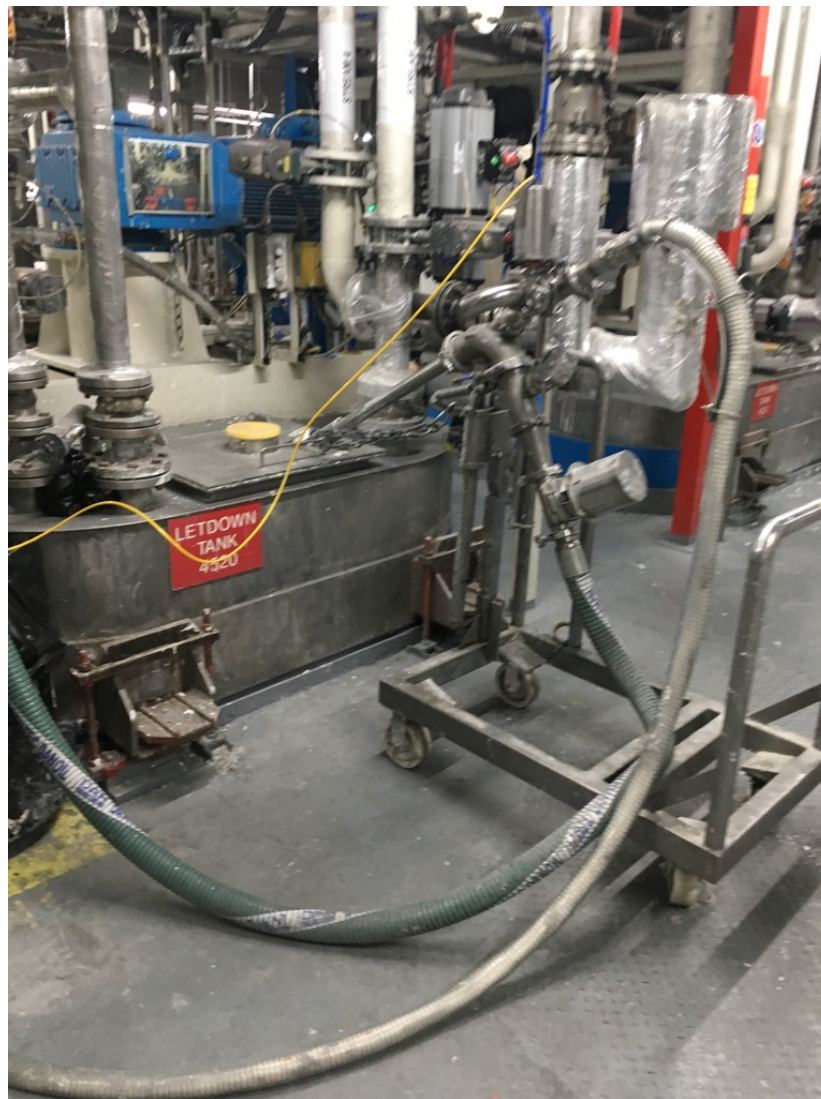
Figure 53: Vessel cleaning at Crown Paints Hull site.
