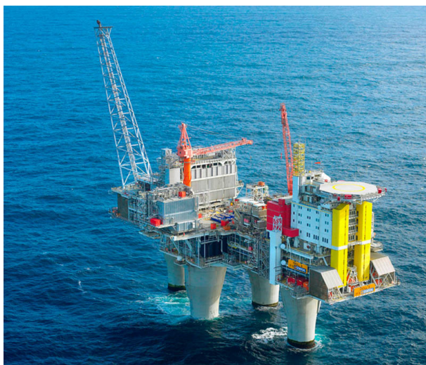
Figure 20. The Troll A concrete gravity base structure (Courtesy: Statoil).
