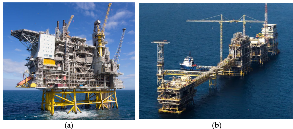
Figure 4. Typical platforms showing (a) conventional jacket platforms and (b) bridged fixed jacket platform on Zuluf oil field in Arabian Gulf, offshore northeast Saudi Arabian coast, with the water depth of about 40 m (Image (b) Courtesy: Saudi Aramco).
