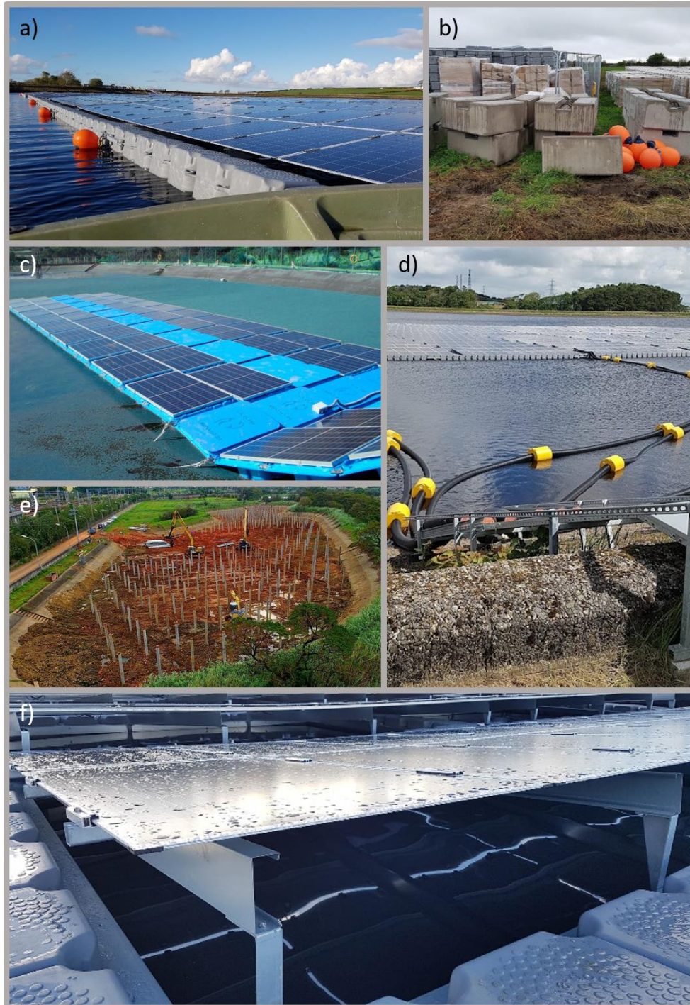
Figure 1-1 – FPV array components. a) a multibody FPV array, b) mooring equipment for the station-keeping system, c) a single-body membrane style flexible floating structure © Isifloating, d) floating cabling to transfer current from the FPV array to onshore balancing equipment, e) an FPV array using fixed mountings built on the bed of the host water body ©Munch, f) the underside of an FPV showing the PV module, HDPE float and the surface of the host water body.
