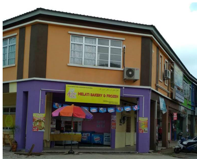
Figure 6.13 Company M after 8 months
