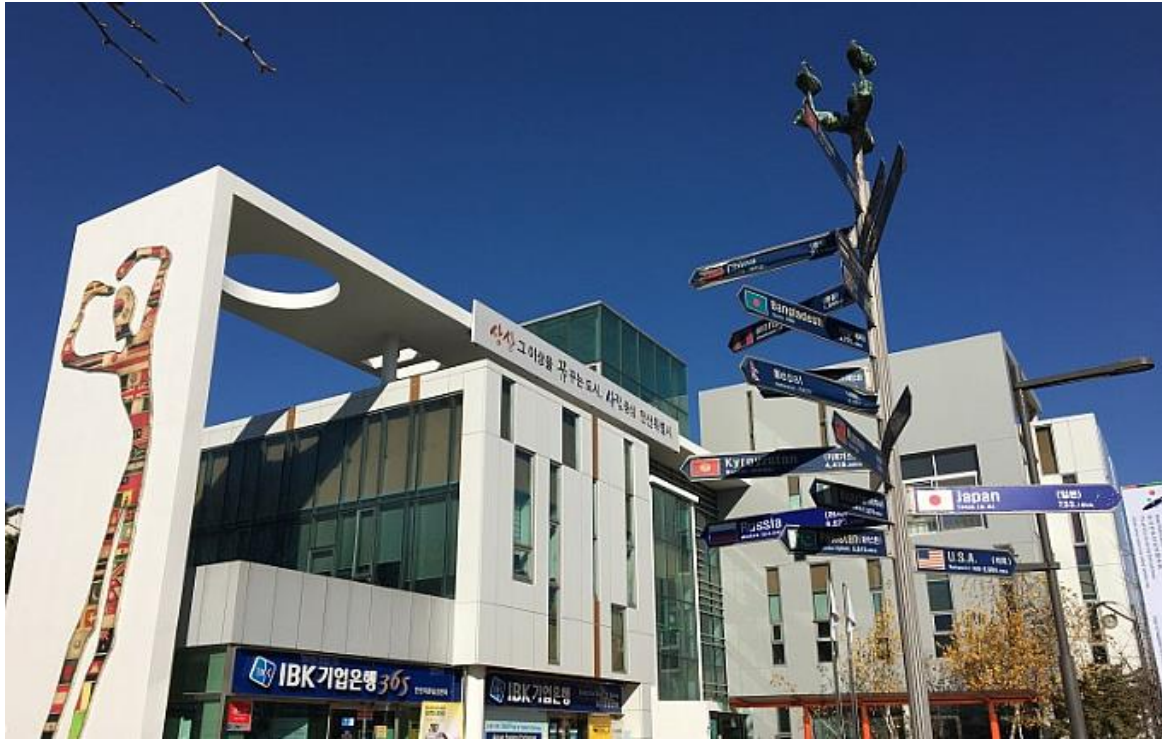
Figure 11. The building containing the AMCSC 61
