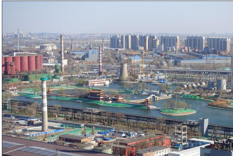
311 Fig. 8 Shougang Park Regeneration Site, Beijing
