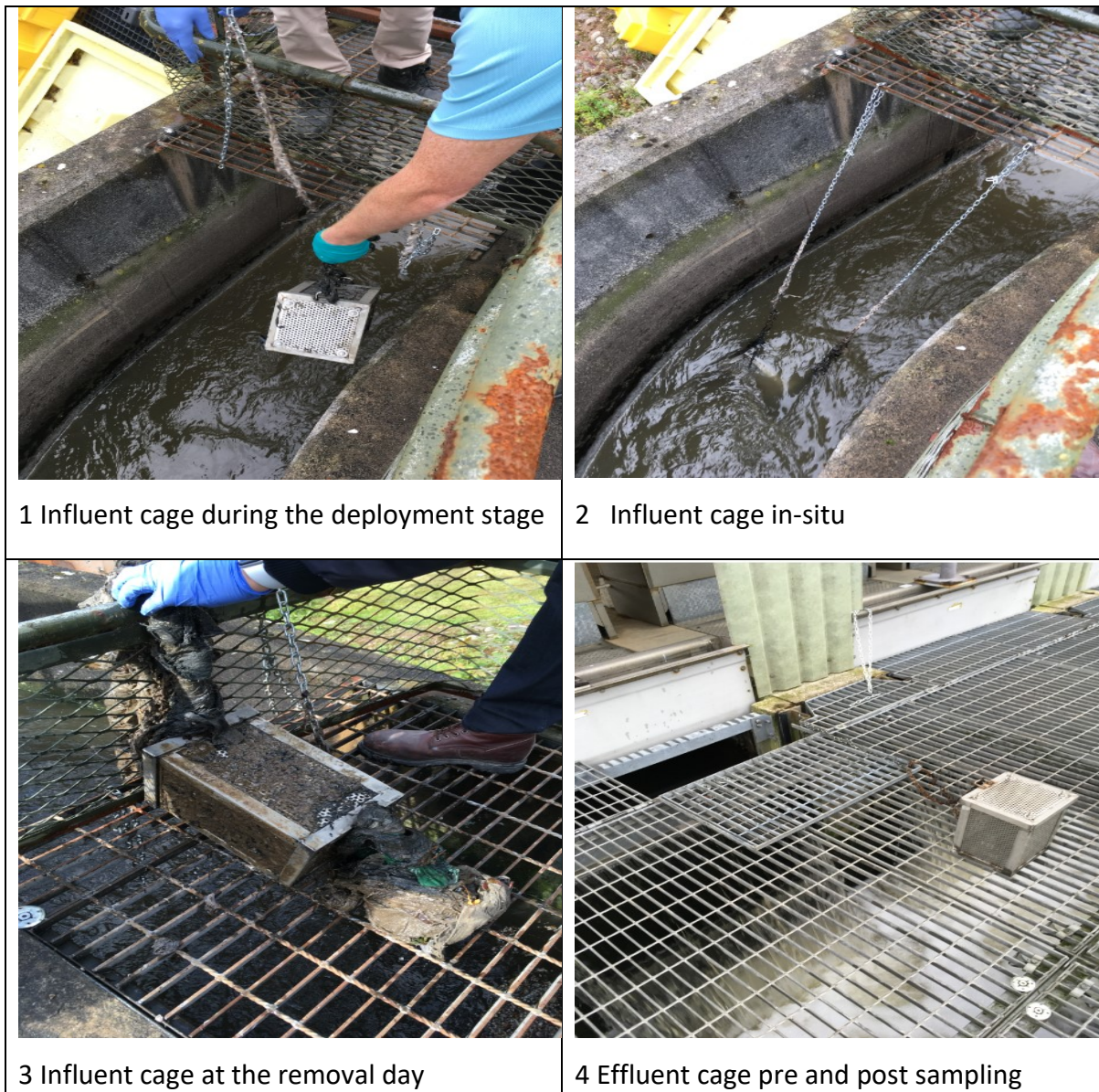
Figure 1: Deployment Device at the influent and Effluent of treatment works
