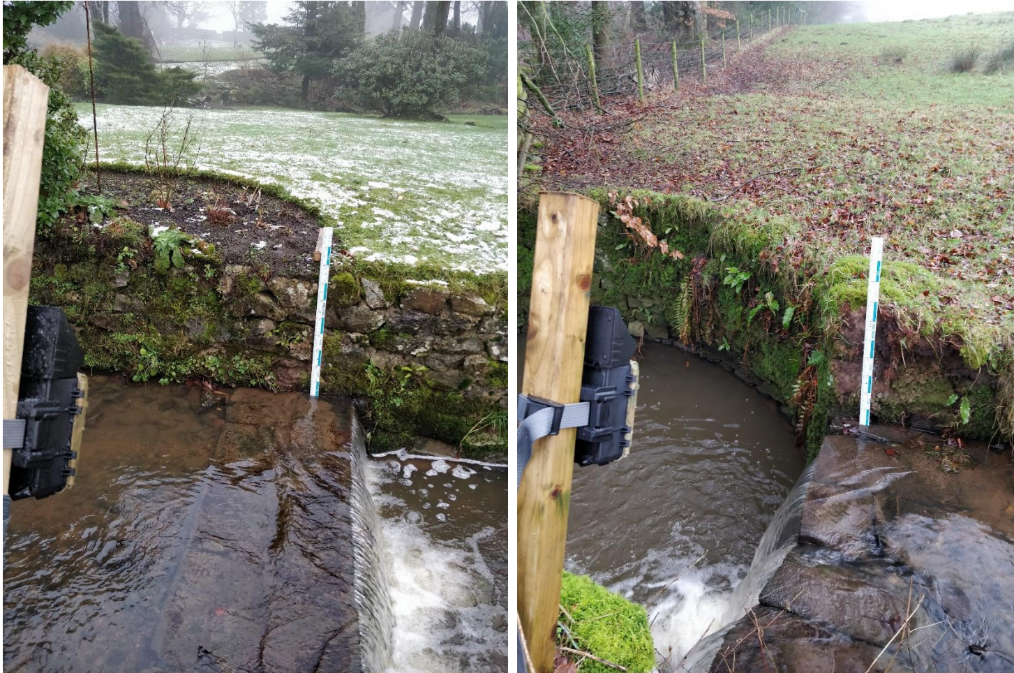
Figure 3.4.1. Photographs of the stage-boards and time-lapse cameras set up at the Mill Brook (Lawn) and Mill Brook (Bull Ring) potential hydropower sites to measure flow depth.
