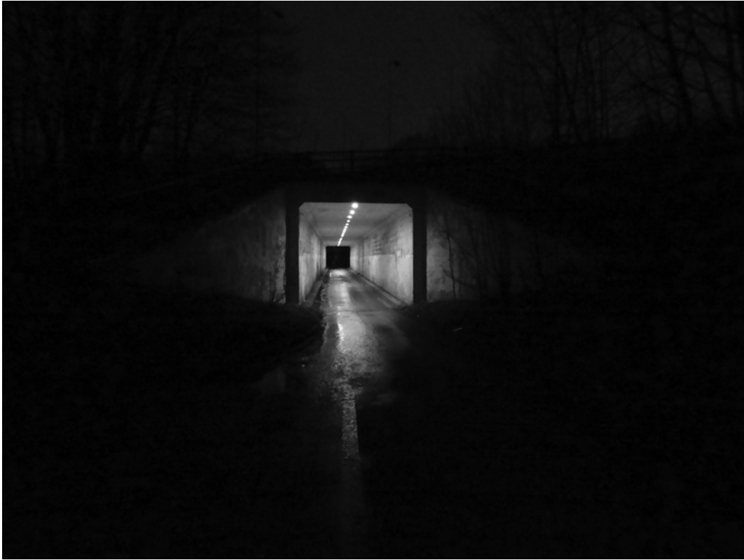
Figure 13.5 M60 motorway underpass, Worsley, 4 April 2018. © Nick Dunn.
