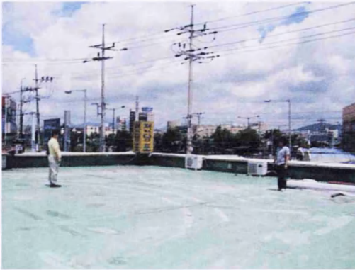
Figure 7.2: YTMP Location, July 2010.
