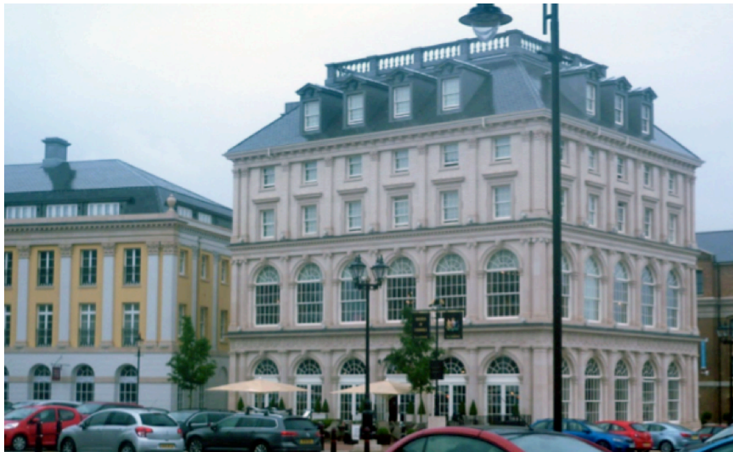
Figure 6.37: 'The Duchess of Cornwall Inn, Poundbury', modeled on London's Ritz Hotel. Photograph by author, July 2017
