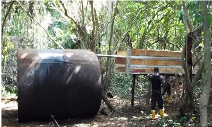
Figure 4.10: Camp operators setting up a refining facility
