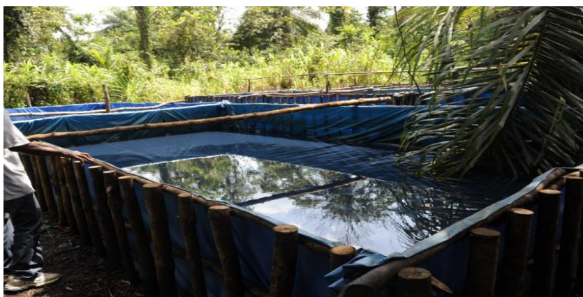
Figure 4.9: A locally made storage facility
