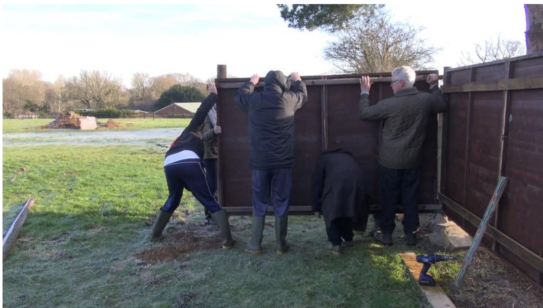
Figure 5.22 Video frame of service users helping to erect a fence
