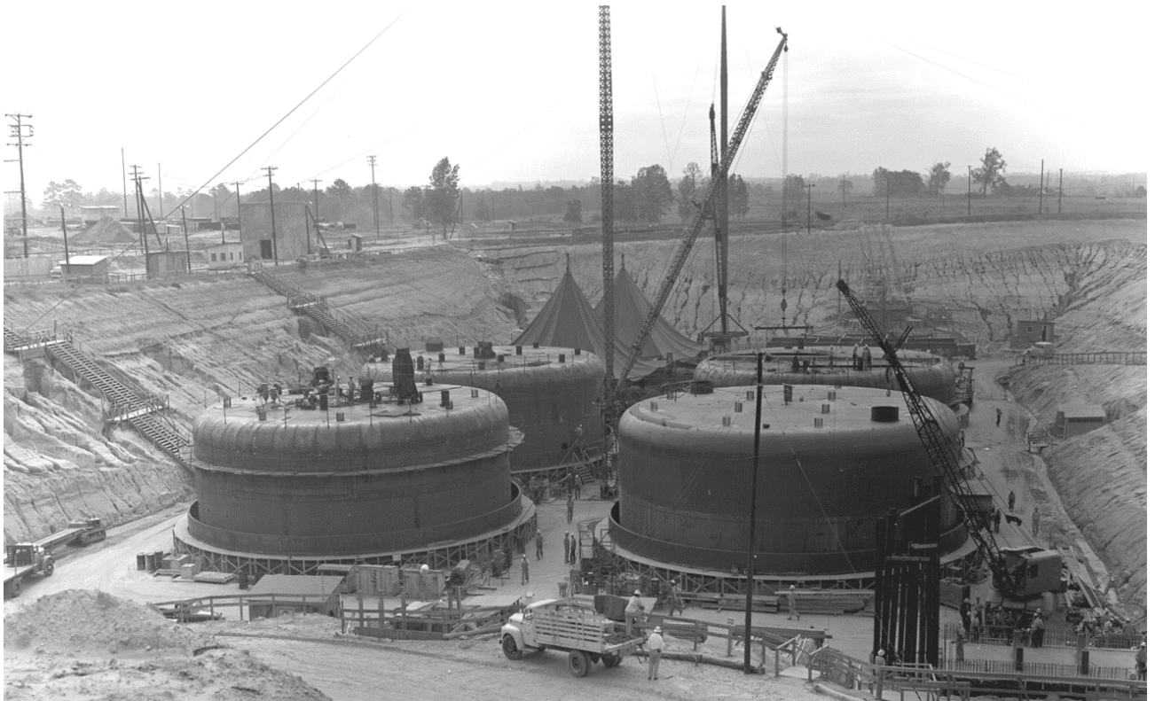
Figure 4. 1950s construction of an SRS HLW tank.
