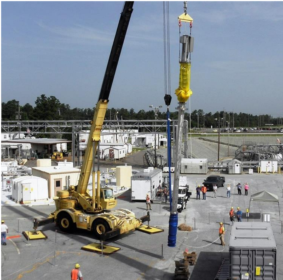
Figure 48. Submersible Mixer Pumps being installed into an SRS HLW tank.
